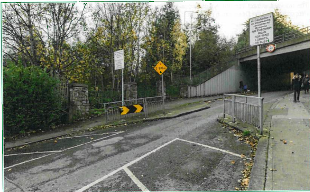
Figure 2.3.8: View from the north – as existing
